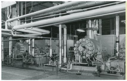
Boiler feed pump for thermal power
